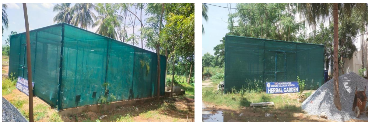
Figure 1: Green House – where the research is conducted
